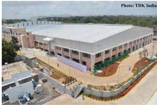
Photo: TDK India Overview of the manufacturing facility of TDK India located at Nashik, Maharashtra.
